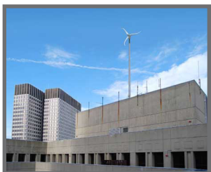
THE WIND TURBINE ON CITY HALL IS A LIKELY EXAMPLE OF A “BUILDING INTEGRATED” WIND ENERGY FACILITY
